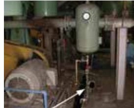
water-cooled after cooler
